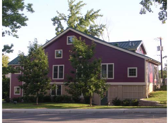
Office Conversion of Historic Barn
